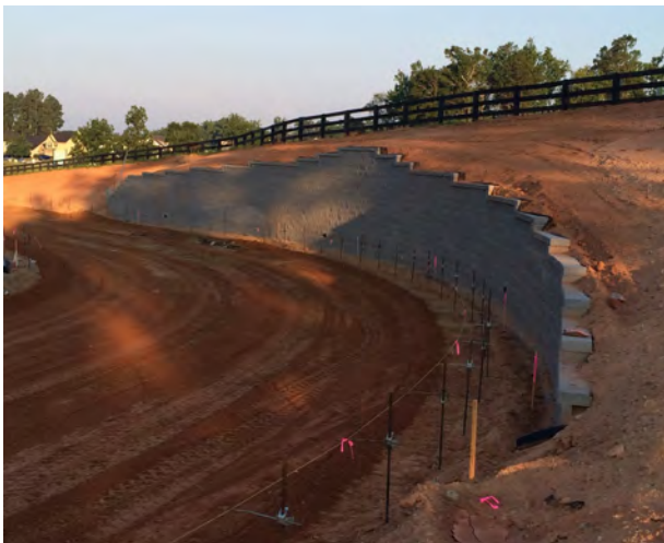
Upper Retaining Wall
