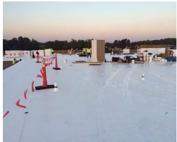
Tower Roof West
