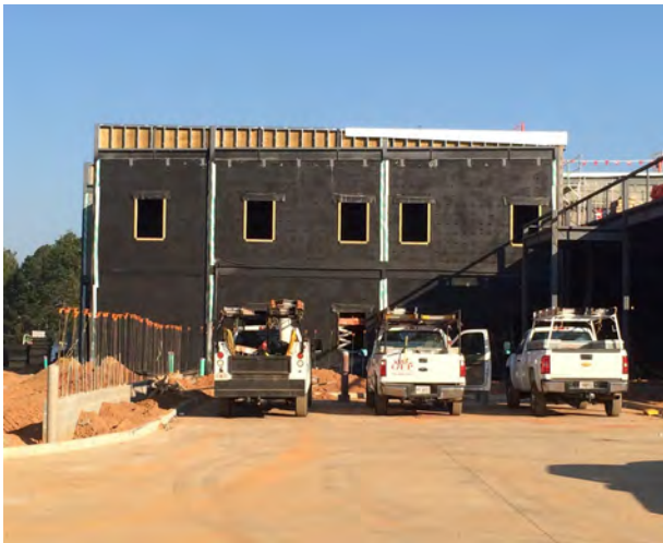
South Tower Elevation West End
