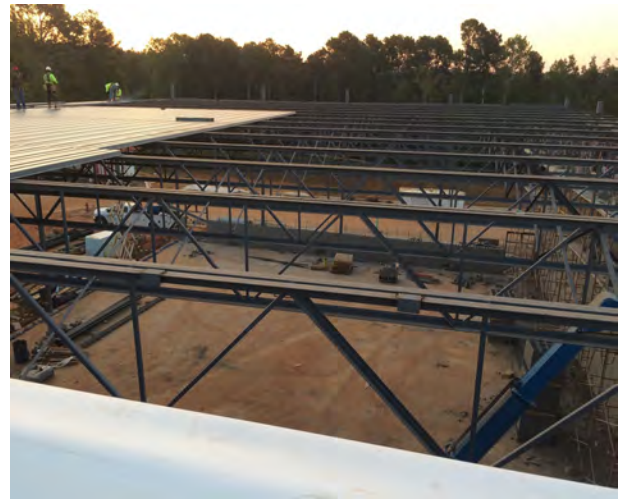
Gym Roof Joists
