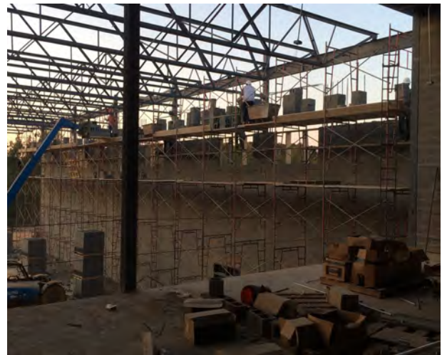
Area D Demising Wall
