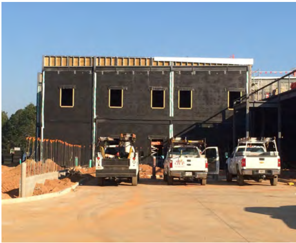
South Tower Elevation West End
