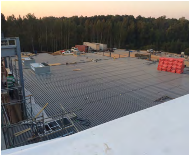
Kitchen - Dining Roof Deck
