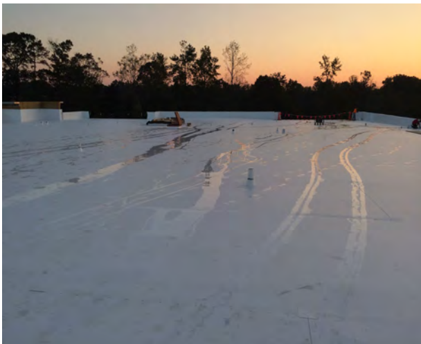
Tower Roof East
